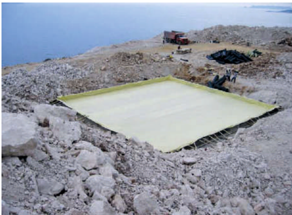
Waterproofing on Lean Concrete
